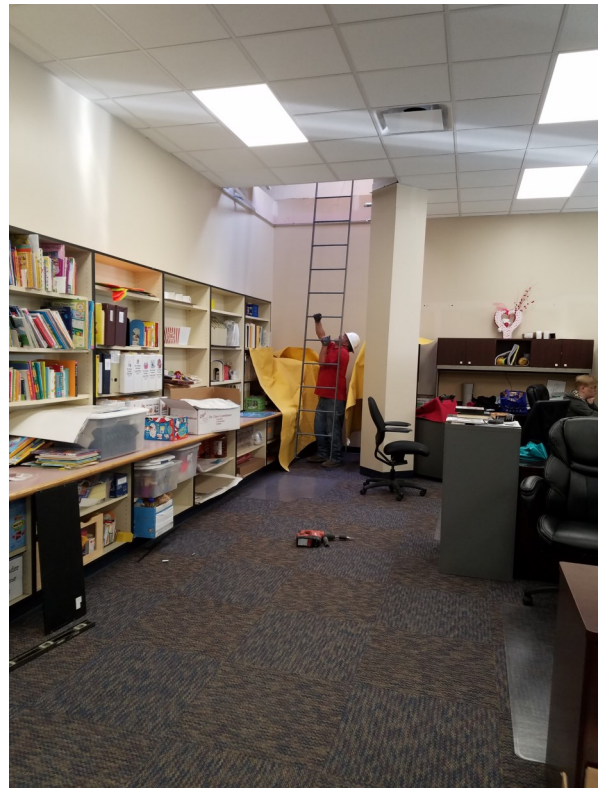
A worker positions a ladder to access space above the ceiling
